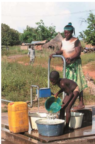
Clean water can be provided by a covered well with a foot pump.
