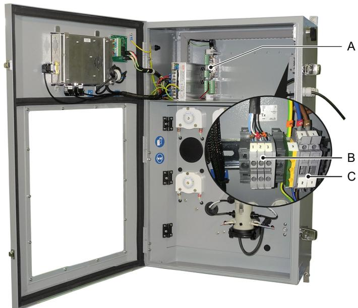
**A** I/O board<sup>1)</sup> (relays, analog signal outputs, digital inputs)
