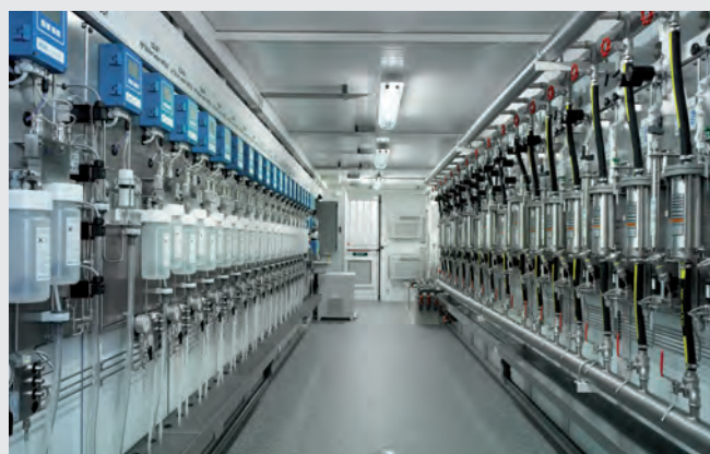
Water / Steam Analysis Equipment for Saudi Electric Company Power Plant PP10 manufactured by SWAN Systeme AG.
